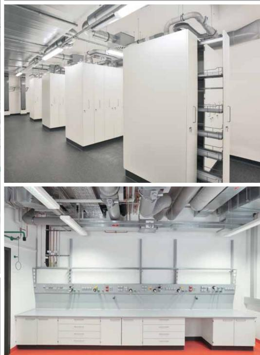
Location: Jena, Germany · Laboratory area: Approx. 3,500 m<sup>2</sup> · Type of laboratory: Chemical and analytical laboratories · Equipment: 200 fume cupboards · Laboratory benches as wall and double work benches · Pull-out cabinets · Special characteristics: Chemical breakdown fume cupboards with integrated fume-
