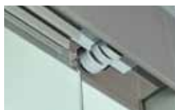
2 Sensors for detector of sash position
